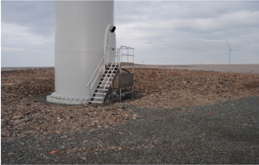
Figure 3. Foundation and tower after backfilling of material (Raggovidda wind power plant).
